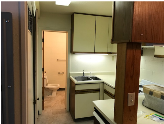
View of bathroom from kitchen
