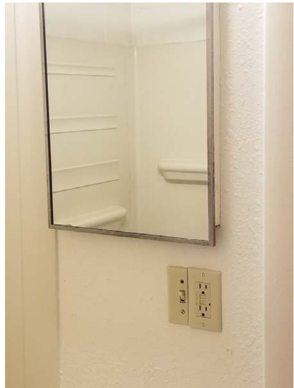
View of mirror and switch/outlet in bathroom
